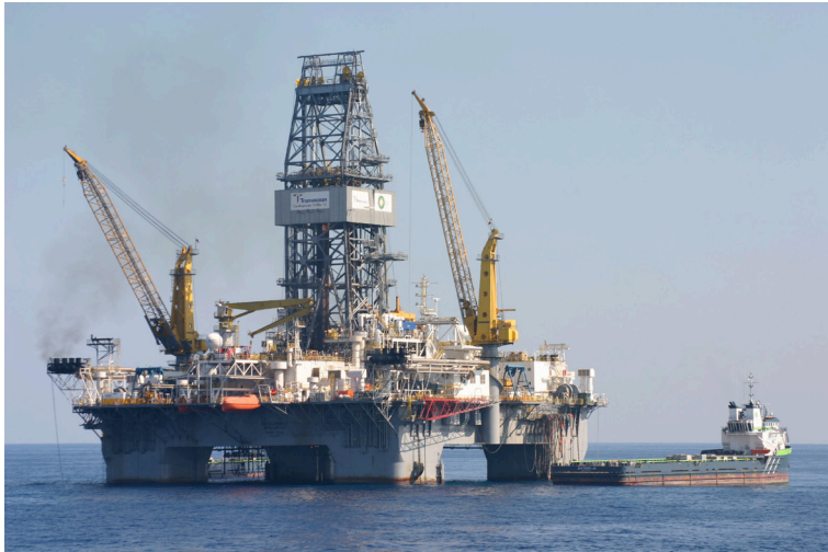
The DD3 drilling rig
